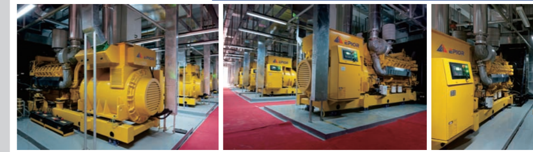
10MW: 2MW*5 sets XDE2500EH3-TX
