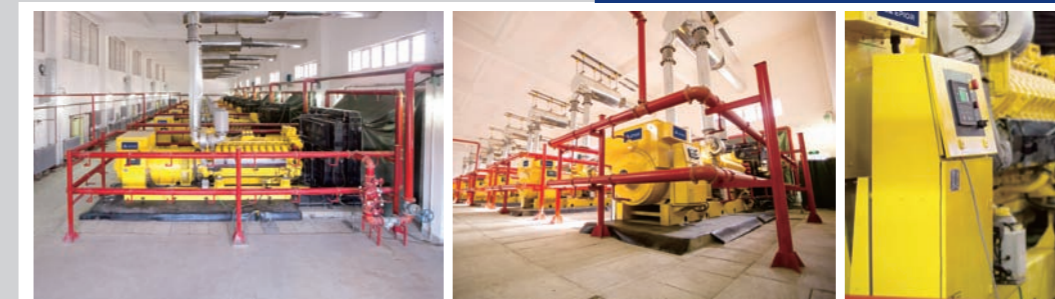
ELECTROLYTIC ALUMINUM THERMAL POWER PLANT 36MW: 2.4MW*15 sets XDE3100EH3
